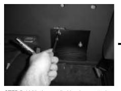
**STEP 5:** With the supplied hardware, attach the bracket to the rear wall.
