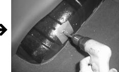
**STEP 5:** With a 1/2" drill bit, drill a hole at the impression on the wax square.
