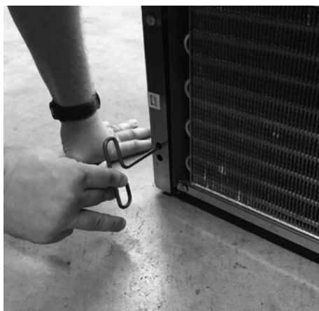
Adjusting rear leveling legs.
