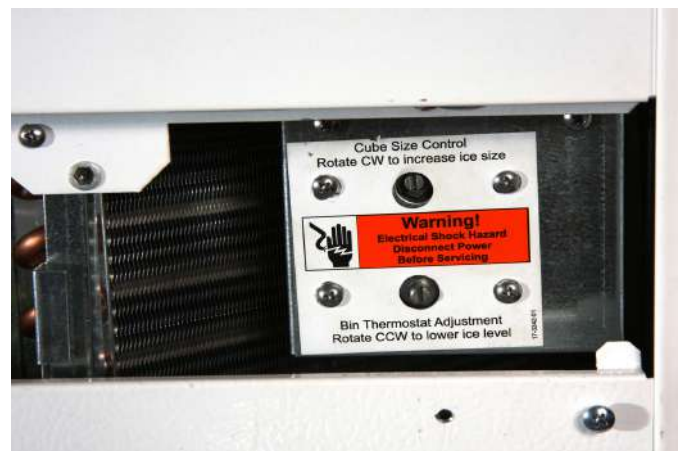
Condenser and Bin Thermostat
