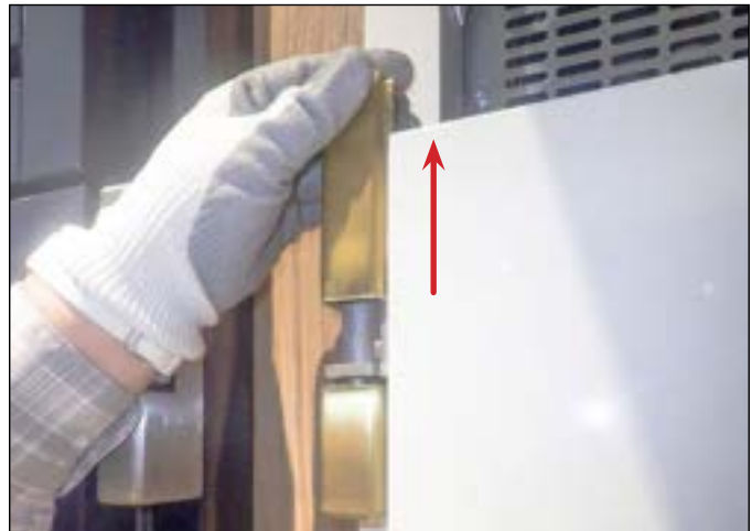
FIG. 2. Remove the hinge covers.
