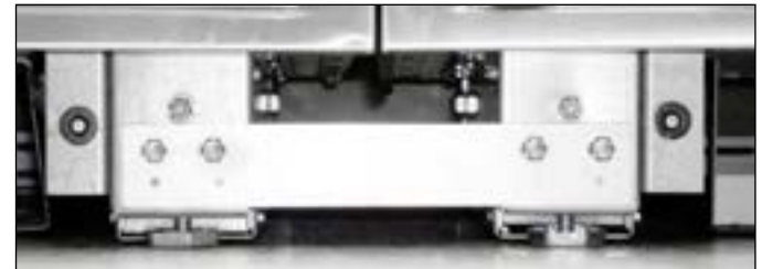
FIG. 18. Installed joining bracket.
