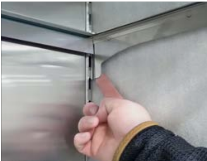
FIG. 6. Push the bottom tab inward.
