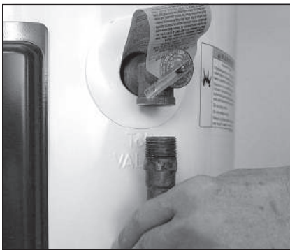
Figure 11 - Removing the T&P Relief Valve discharge pipe.
