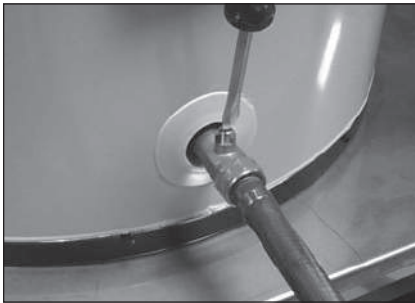
Figure 10 - Draining the old water heater.
