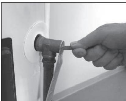
Figure 41 - T&P Relief Valve
