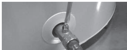
Figure 29 - Drain Valve
