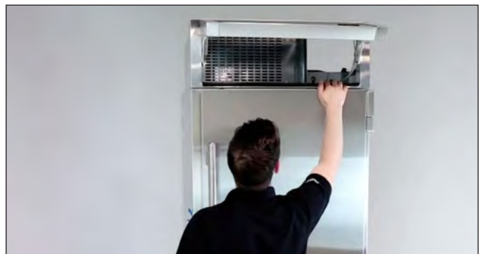
FIG. 3. Be sure to inspect the rainshield.
