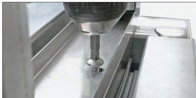
FIG. 10. Remove the screws from the metal channel.
