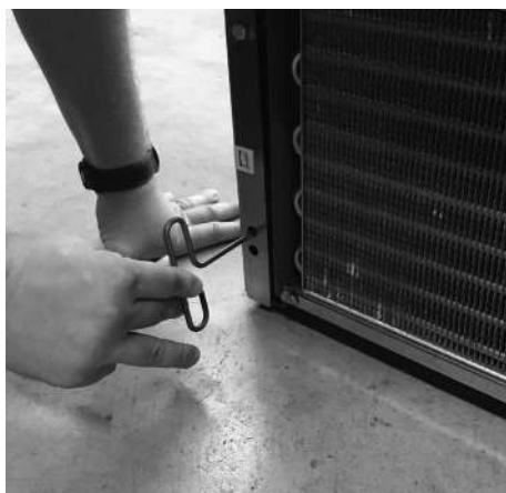
Adjusting rear leveling legs.
