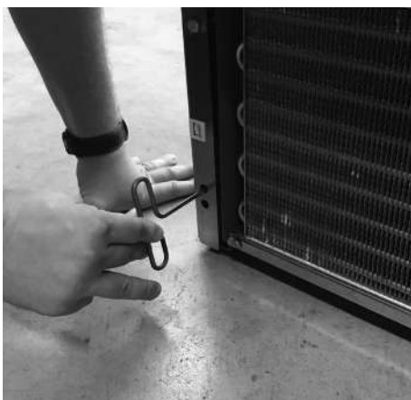
Adjusting rear leveling legs.
