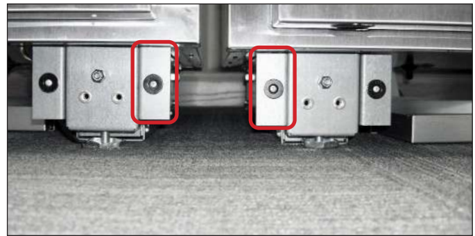
FIG. 11. Remove and discard the interior magnet brackets.
