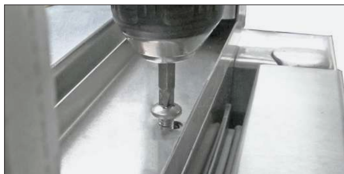
FIG. 10. Remove the screws from the metal channel.
