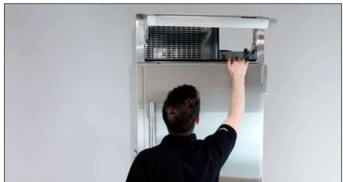
FIG. 3. Be sure to inspect the rainshield.
