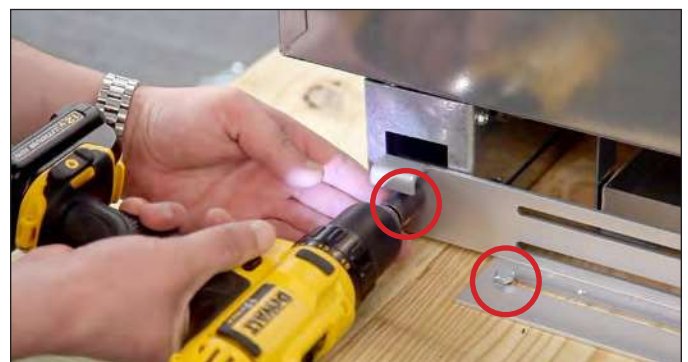
FIG. 8. Anti-tip bracket shipping bolt locations. Other side not shown.
