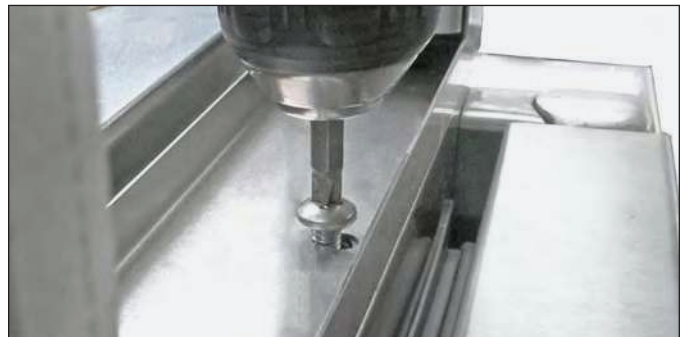
FIG. 10. Remove the screws from the metal channel.
