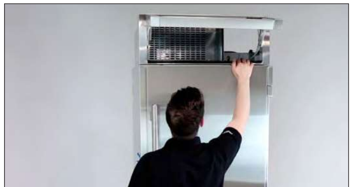
FIG. 3. Be sure to inspect the rainshield.
