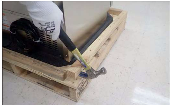
FIG. 2. Pry the side runner board off the skid.
