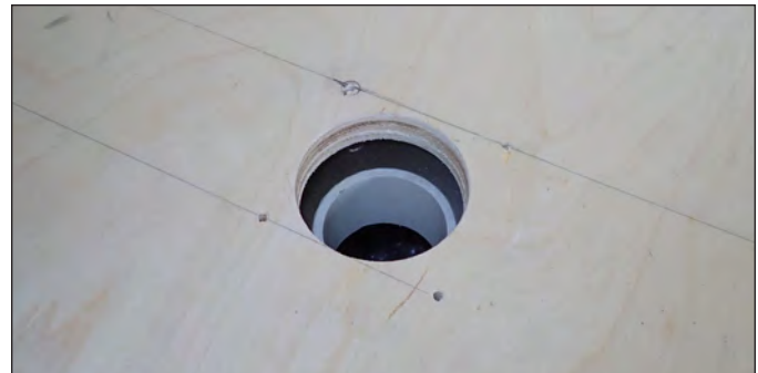
FIG. 4. Align the holes in the appliance with the drilled hole.
