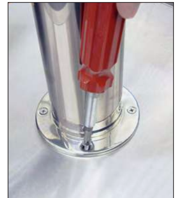
FIG. 3. Secure the draft standard to the countertop.
