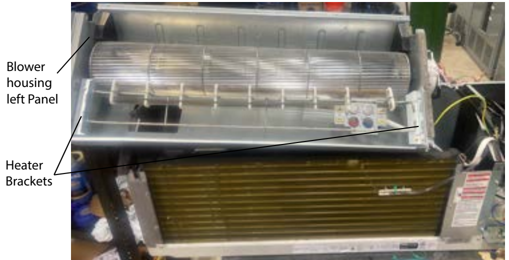
Figure 710 (Slide up Housing)
