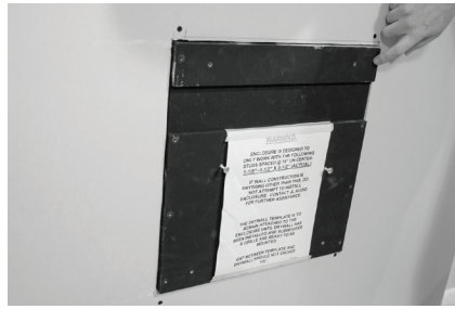
Figure 25 Install surrounding wallboard flush against wallboard template.
