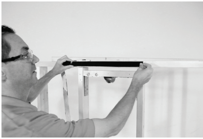
Affix foam gasket strip to all stud and mounting bracket faces.
